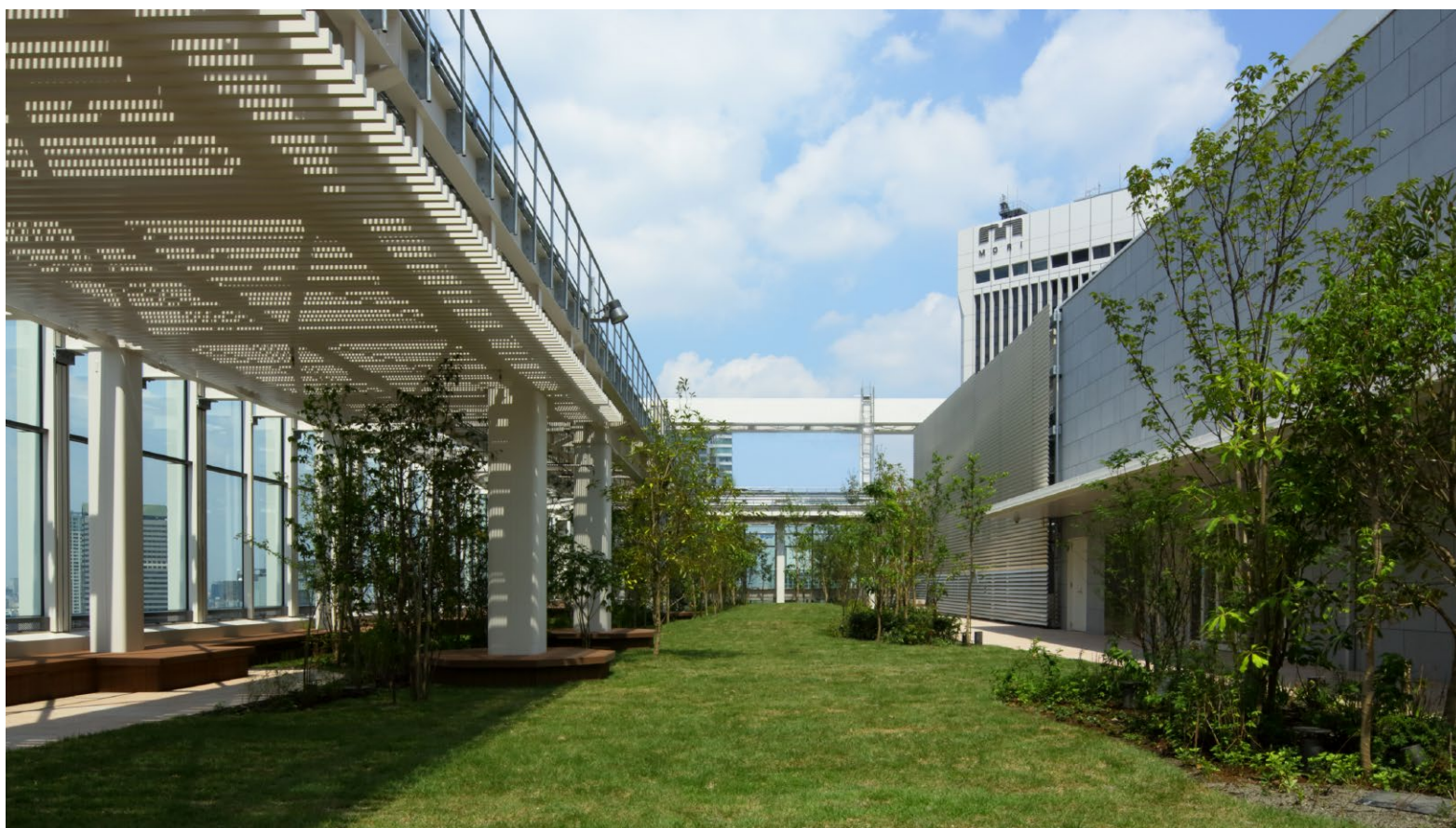
▲ Roof Garden "Sky Park"
